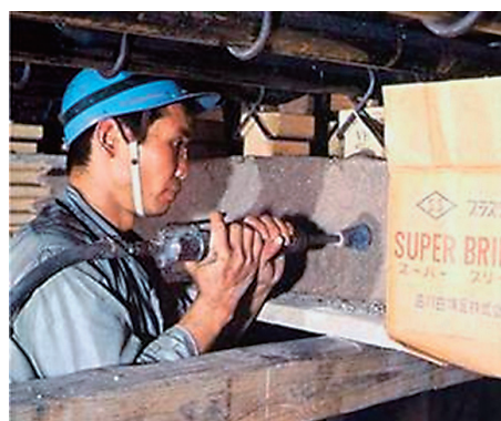
Fig. 2 Scene of ramming plastic refractory installation onto wall surface.
