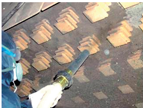
Fig. 4 Scene of gunning plastic refractory installation onto wall surface.
