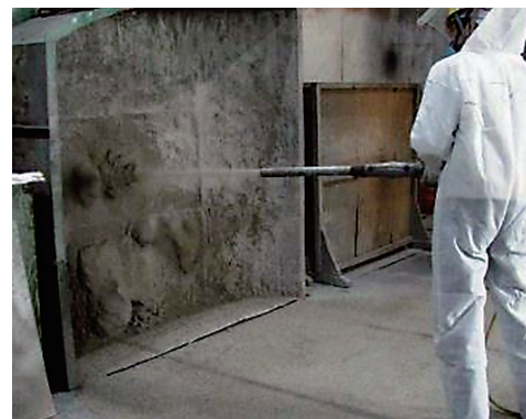
Fig. 10 Scene of gunning experiment of dry-gunning repair refractory material.
